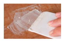
Step-2 Fill Holes and cracks with Putty Paste
