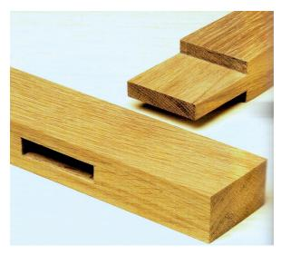
Fig 3.1.6.1: Mortise and Tenon Joint
