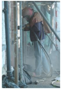
Fig 10.3.2: Abrasive Blasting
