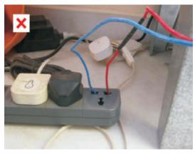
Fig 9.2.3.3: While working with power tools, don't plug in the tools haphazardly
