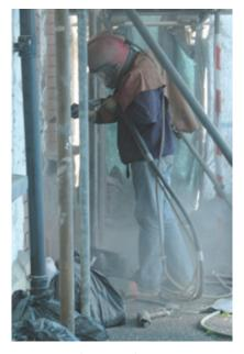
Fig 7.3.2: Abrasive Blasting
