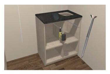
Fig. 1.4.45: Place the counter top on the cabinet
