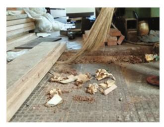
Fig 5.3.1.15: Collect waste from different parts of the workplace
