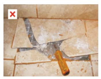
Fig 9.2.3.5: Use floor guards; not using floor guards may damage the floor
