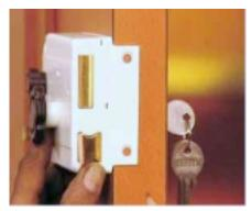
Installation Position of Rim Lock on Door
