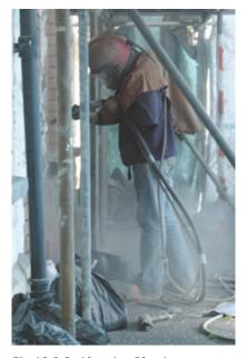
Fig 10.3.2: Abrasive Blasting
