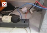
Do not put wires directly into socket; use plug
