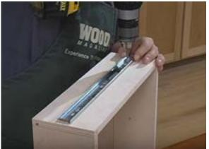
**STEP 4:** First drive the screws into the first and last holes, and then finish by driving rest of the screws. Make sure that the screws are mounted flush with the steel surface to prevent any sticking or catching
