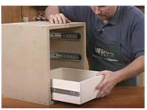
**STEP 12:** Slide the inner member attached to the drawer into the outer member attached to the carcass and close the drawer. The drawer slide release lever will automatically lock as the drawer is closed.
