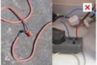
Do not use broken sockets and plugs or frayed wires
